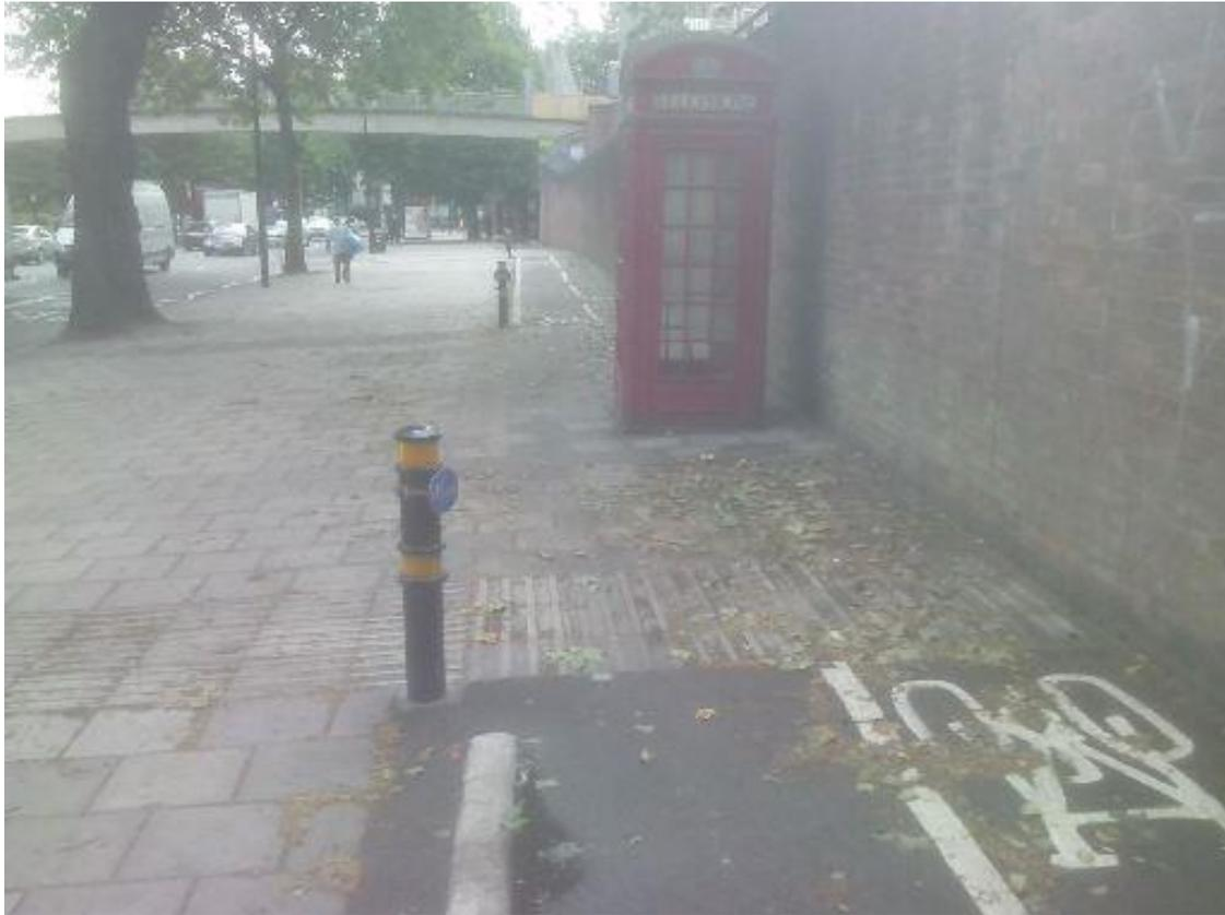
Photo 10: looking eastbound. The segregated use sign (which is presumably aimed at westbound cyclists) is facing the wrong way, but also has the cycle track and the pedestrian area shown the wrong way round.
