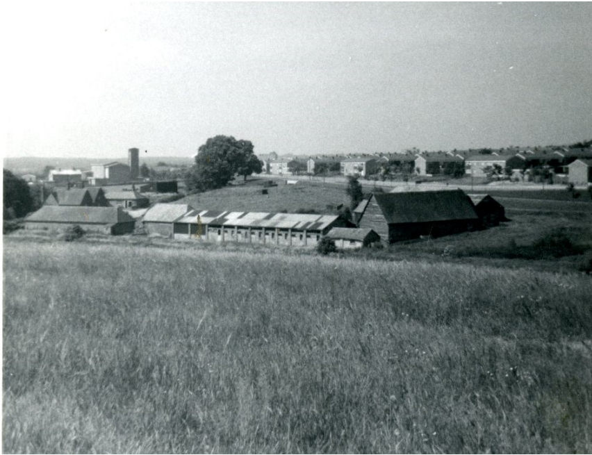
Fairlands Farm buildings from the south 1971
