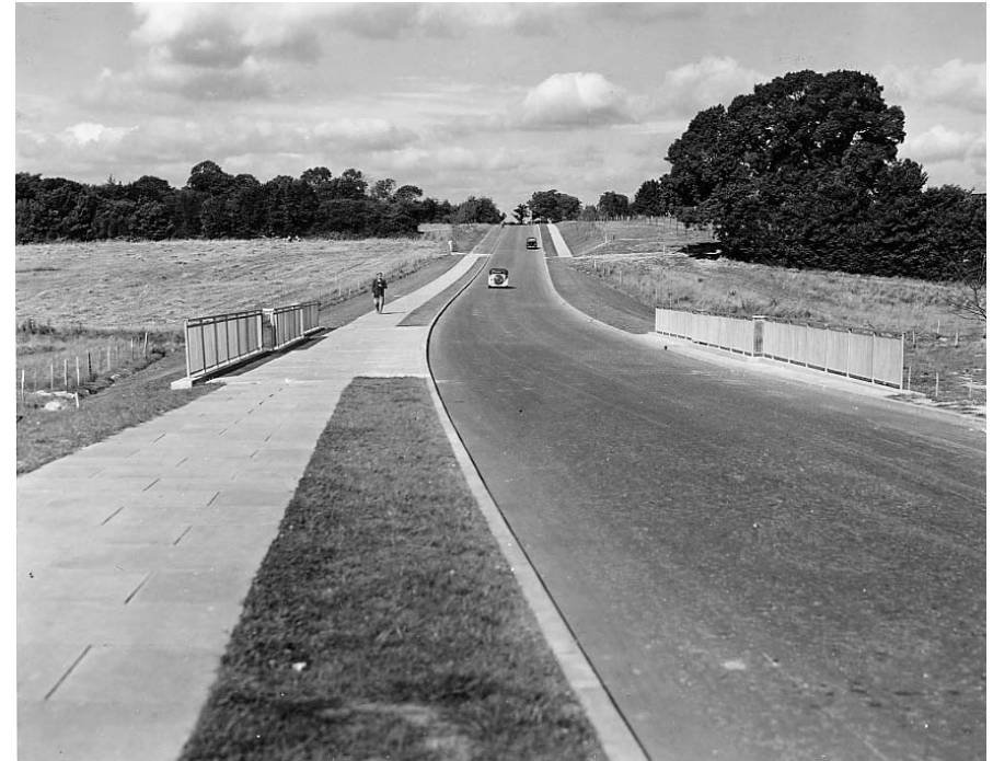
View of Six Hills Way at Fairlands Valley 1955
