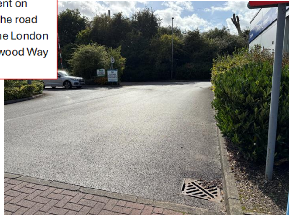
2 – Pedestrian route joining carpark across entrance road without dropped kerbs
