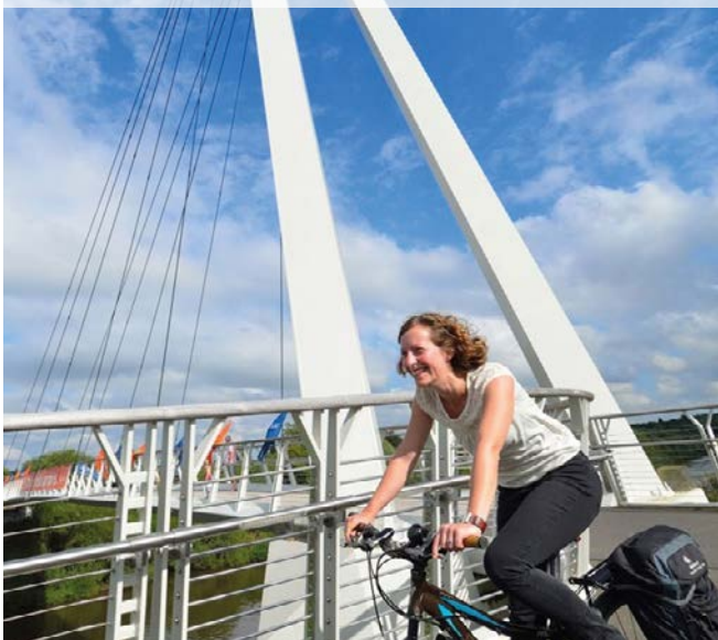
Figure 10.49: Diglis Bridge, Worcester
