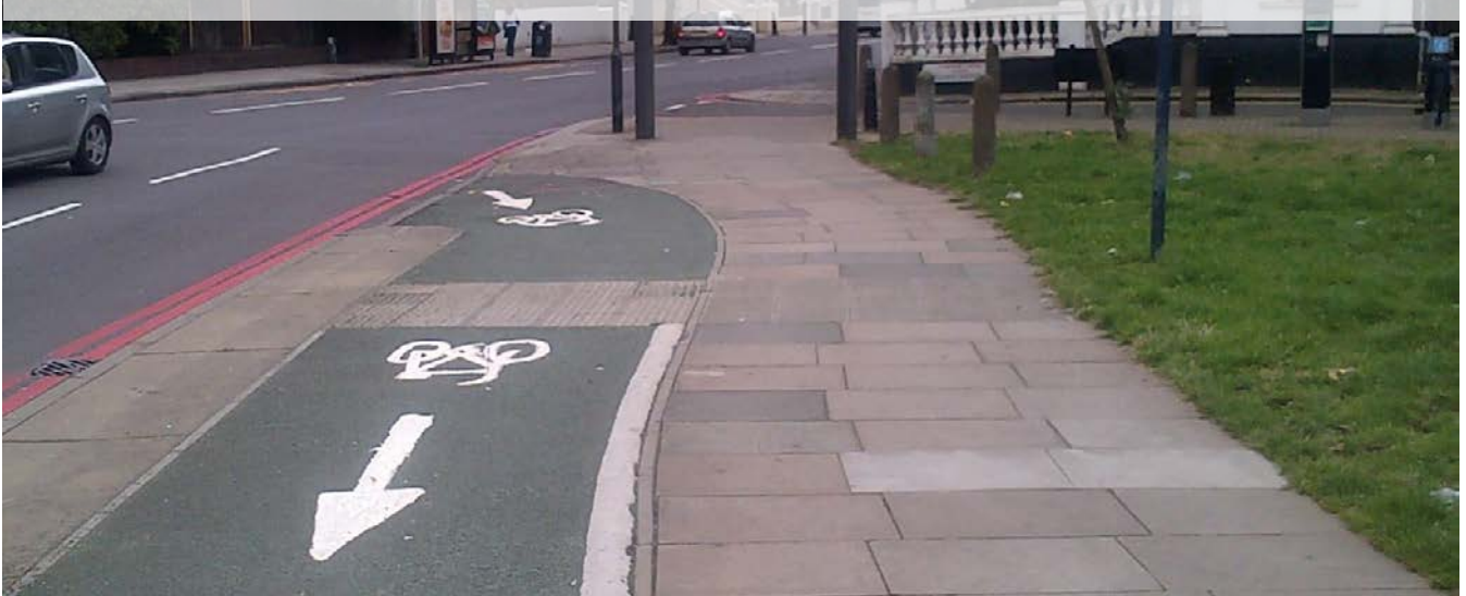
Figure 9.7: Use of arrows to direct cyclists to off-carriageway route, Shepherds Bush
